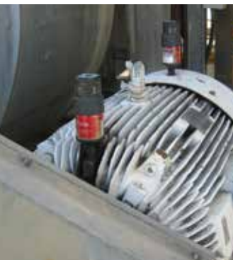
Drive motor lubrication (2 points)
