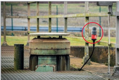
Aeration tank: Lubrication of bearing at surface aerator
