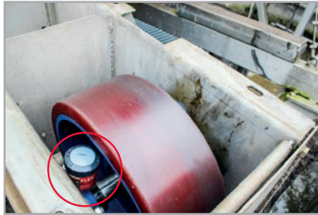
Grit and grease removal: Lubrication of flanged housing units at the scraper
